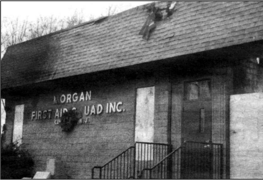
The Morgan First Aid Squad, which recently completed extensive renovations, was completely gutted by a huge electrical fire. Notice the scorched area from flames on upper left and also damage in center, windows and doors are also boarded up. The building will have to be demolished. (Photo by Tom Burkard)
