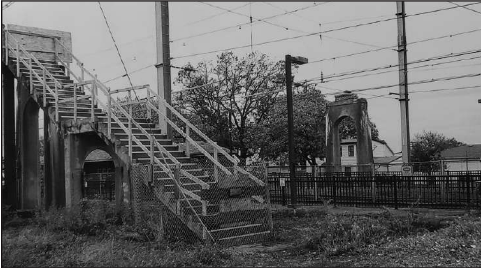
The following day, the bridge has been demolished, and all that remains is pieces and steps which have not been taken down.
