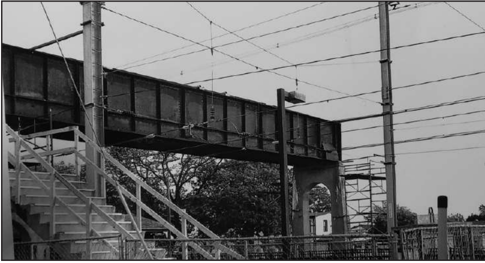
This is the remains of what the old Henry St. foot-bridge looked like on Oct. 25th. The structure was built in the late 1920's and early 30's.
