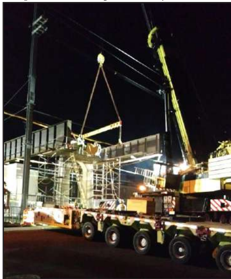
Cranes and other equipment is used to dismantle the old footbridge on Henry St. (Photo by Joann Niestempski)
