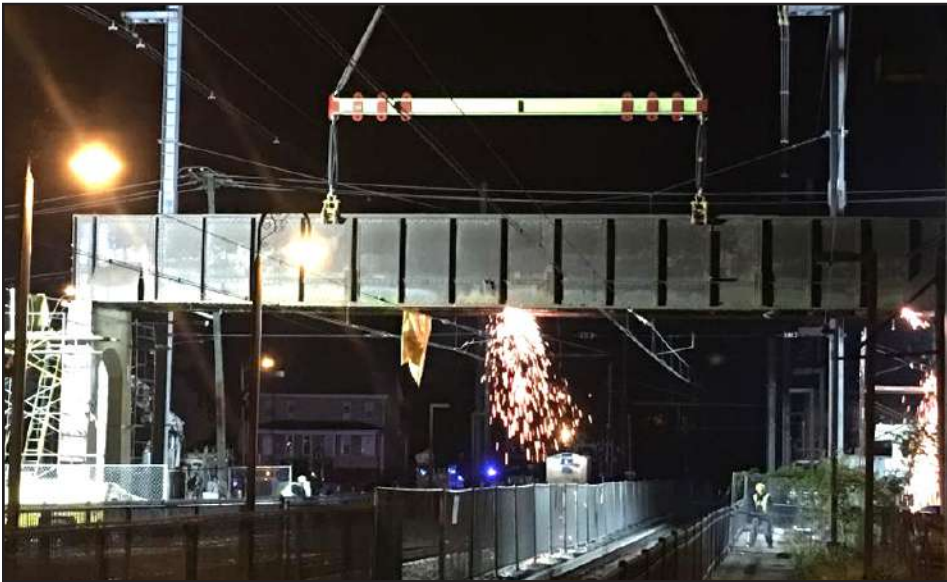
Sparks fly on the railroad tracks while demolition takes place on the bridge. (Photo by Don Zrebiec)
